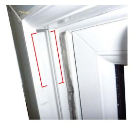
From both sides of the retaining groove measure back 5mm and mark the frame
