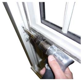
Remove the screws securing the springs
