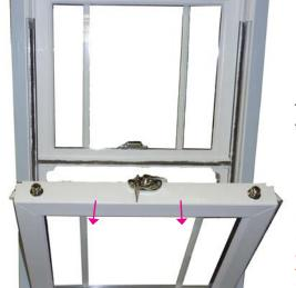
Tilt sash inwards to allow access to the tilt restrictor arm
