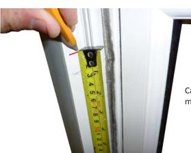
Carefully measure 20mm up from the pencil line and mark the outer frame
