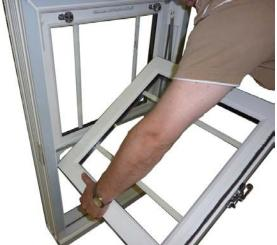
Once one side of the sash has been disengaged from the shoe this will then allow the other side of the sash to also be disengaged and the sash removed.
