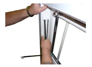
Use a screwdriver or similar to carefully prise the clip fit sash stop from it's location groove.
